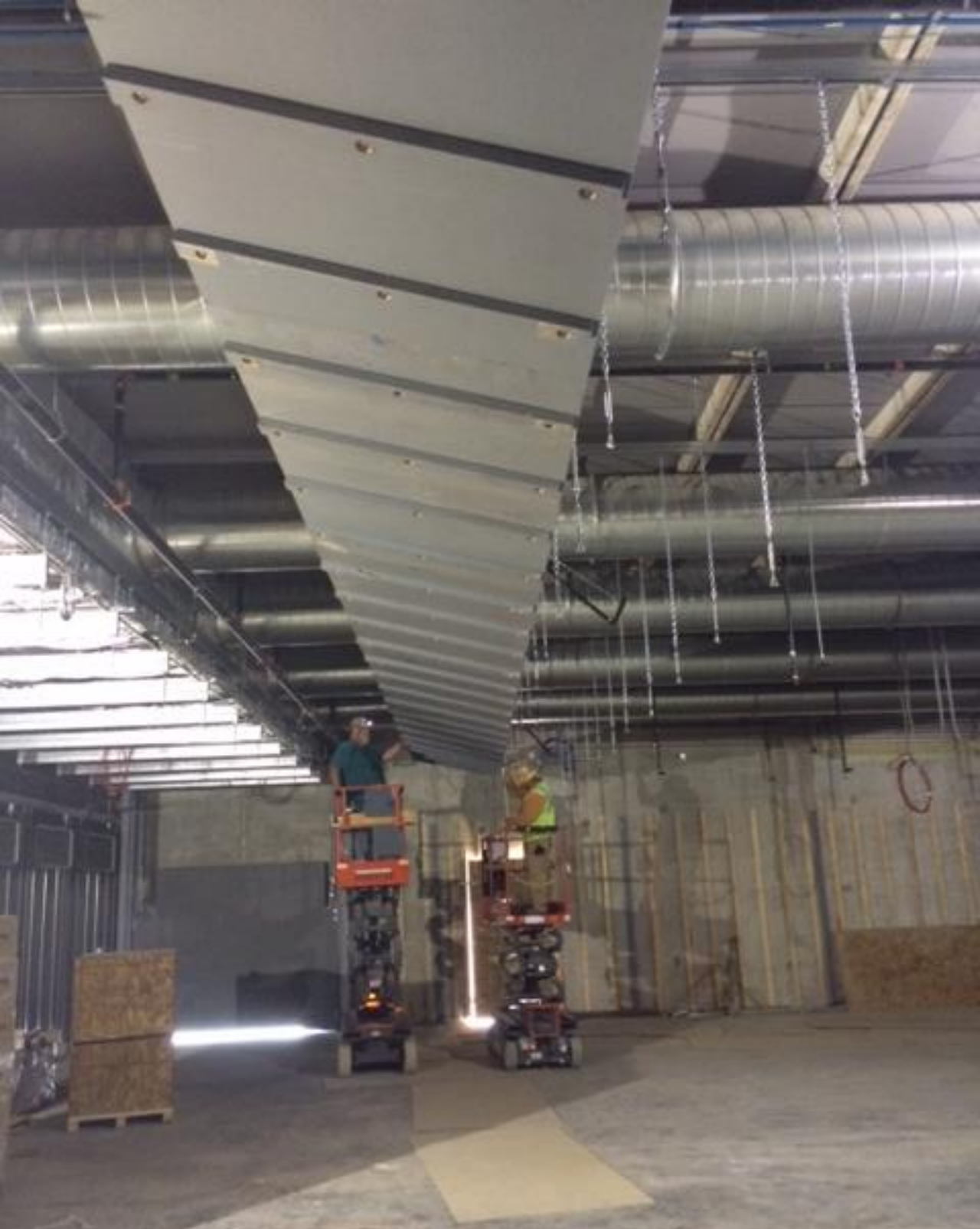
Installation of Angled Baffles in Range on 5/21/15
