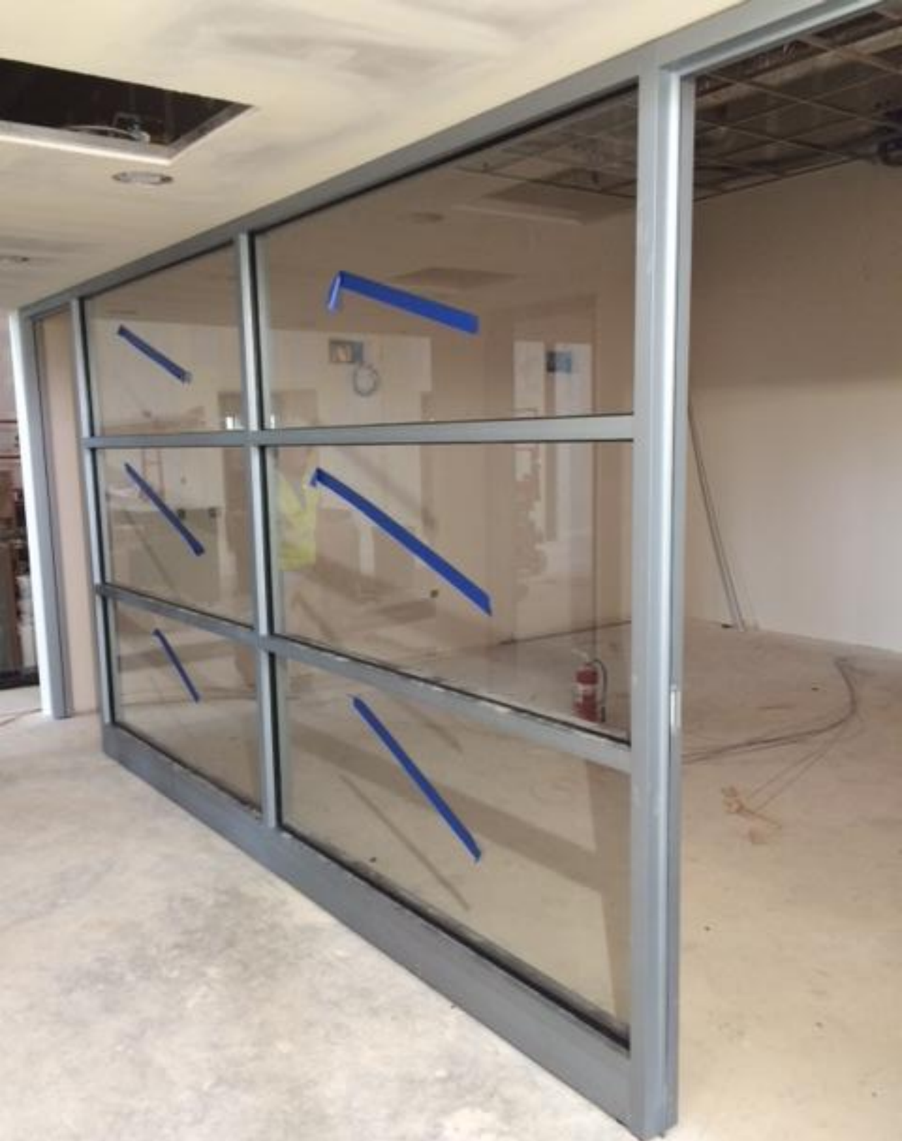
Conference Room Storefront Glazing on 5/15/15
